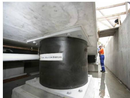
Figure 74 Base Isolation
