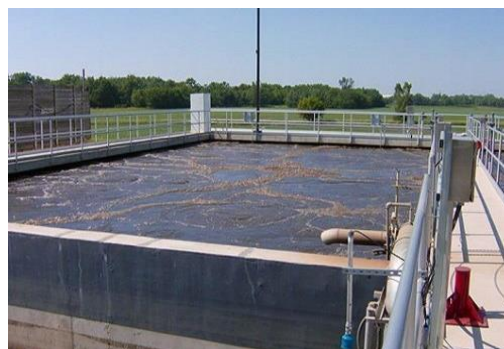
Figure 42 Sewage Treatment Plant
