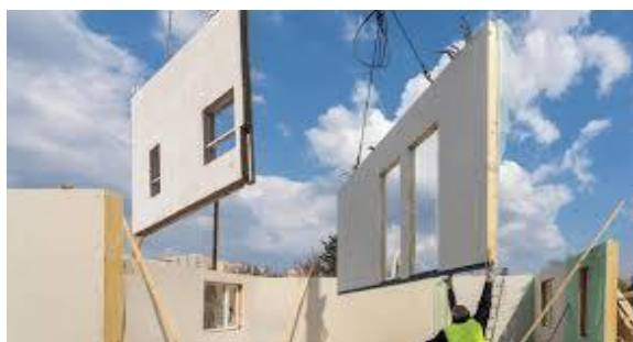
Figure 34 Modular Construction Techniques
