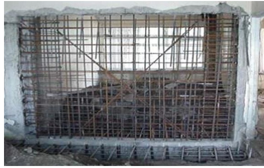
Figure 75 Additional Shear Wall
