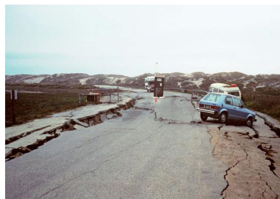
Figure 36 Soil liquefaction
